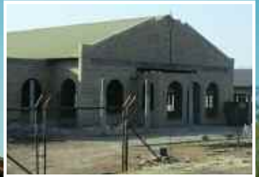
A new Seventh-day Adventist church is under construction in Gaborone, Botswana.
